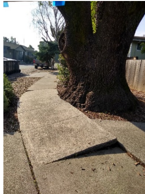
Fig. 5. 2019/2020 Grand Jury. Another displaced sidewalk not listed on the sidewalk service list. 2020.
