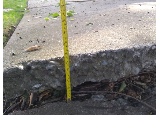
Fig. 4. 2019/2020 Grand Jury. Close-up view of the same sidewalk as Fig.3, showing a displacement of nearly 6 inches. 2020.
