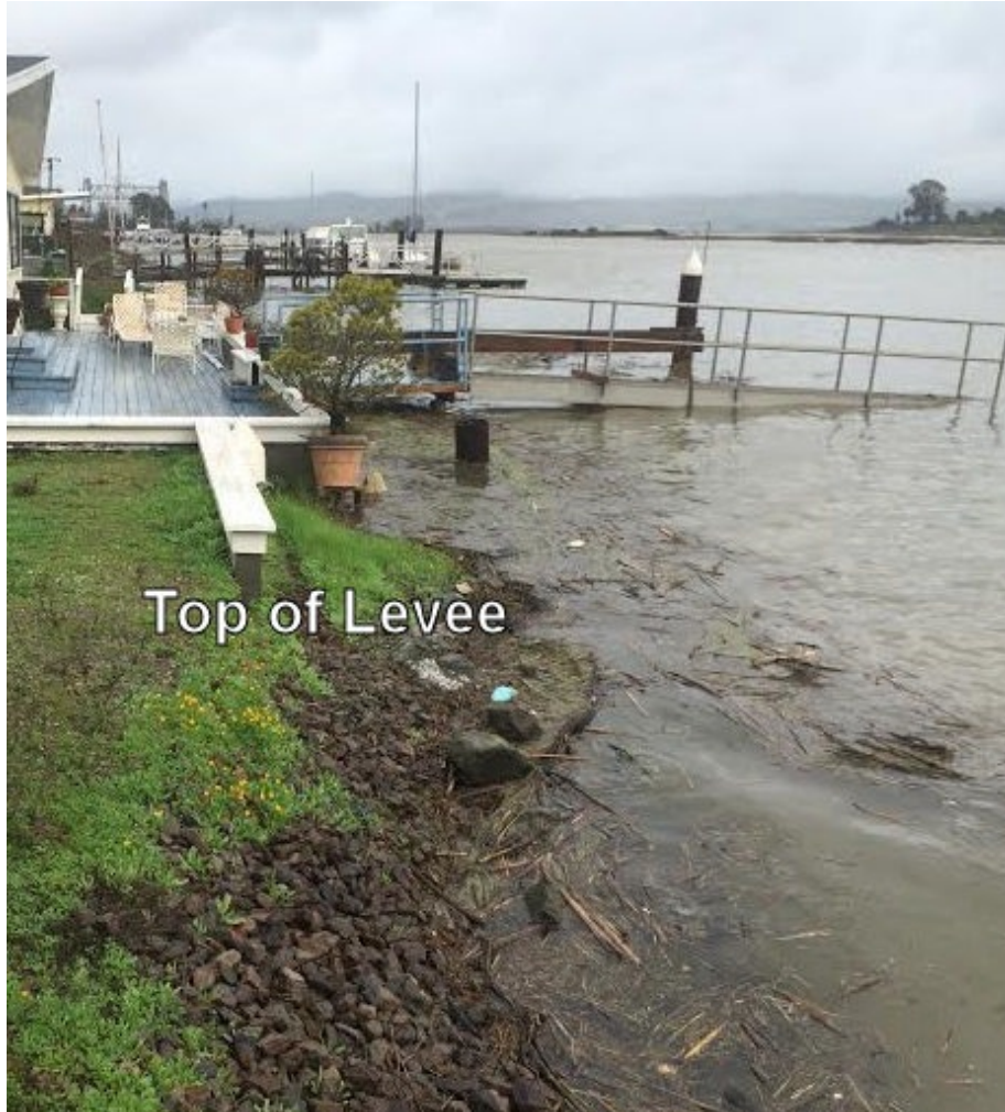
Note the partial submersion of a boat pier and the overbuilding of the levee with piers and a home's deck.
