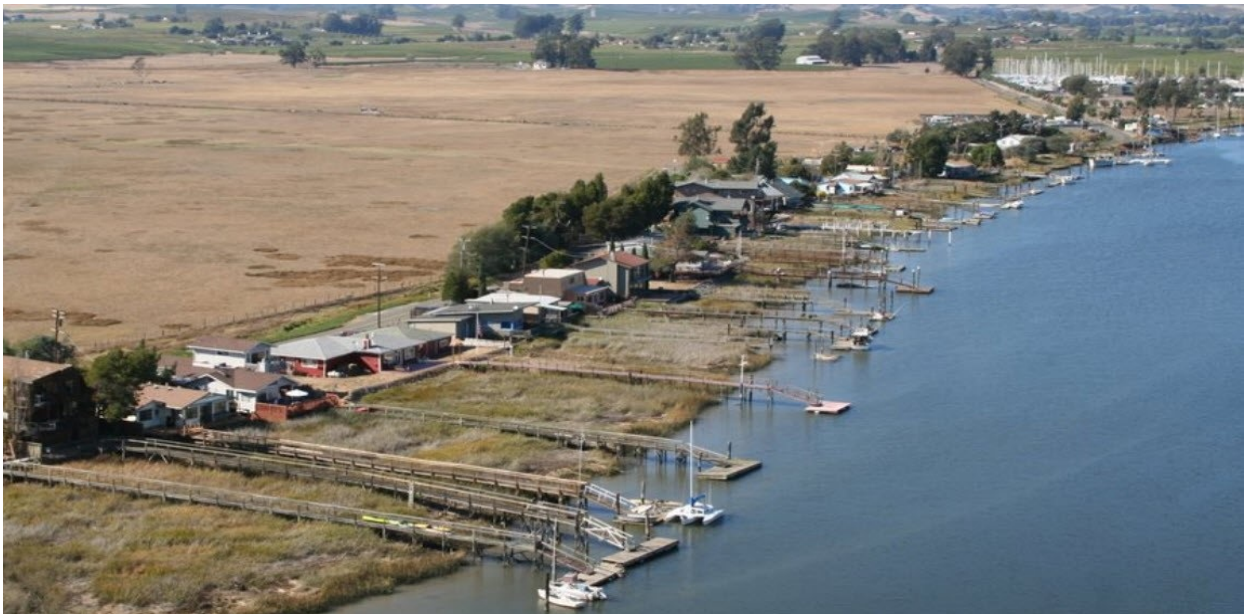
Figure 3. Levee Access Restricted by Boat Docks and Piers
